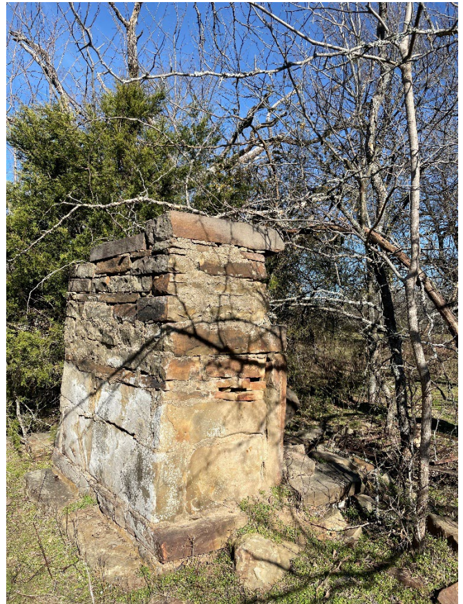
Old chimney at Brushey Jim's, 2023
